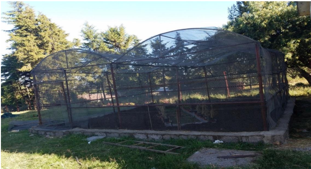
Fig.32. Aditonal Lath-house constructed at KARC
