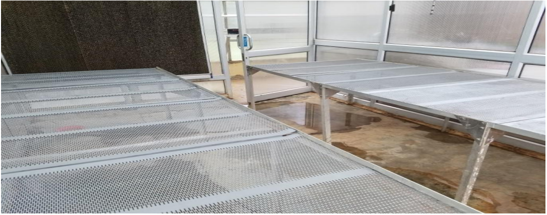
Fig. 33. Greenhouse benches renovated
