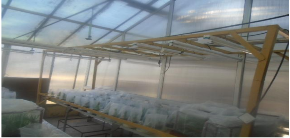
Fig. 31. Green house facilities renovated
