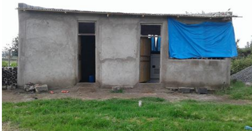
Fig. 48 Green houses and Generator room
